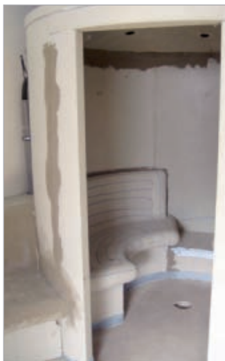
■ Detailed view of the bench: Curved shapes are possible without any problems using the moisture-proof hard foam support elements.
