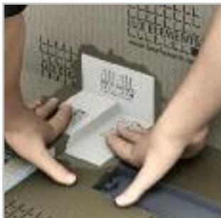
DRY-DBIE LINE – sealing tape for inner corners, for TUB-LINE with single-sided gradient
