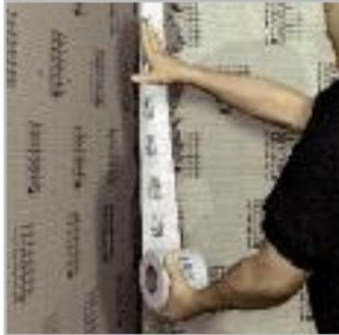
DRY-DB(V) – integrating sealing tape into wall/floor connections
