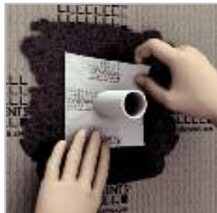
DRY-DBWM – sealing pipe duct
