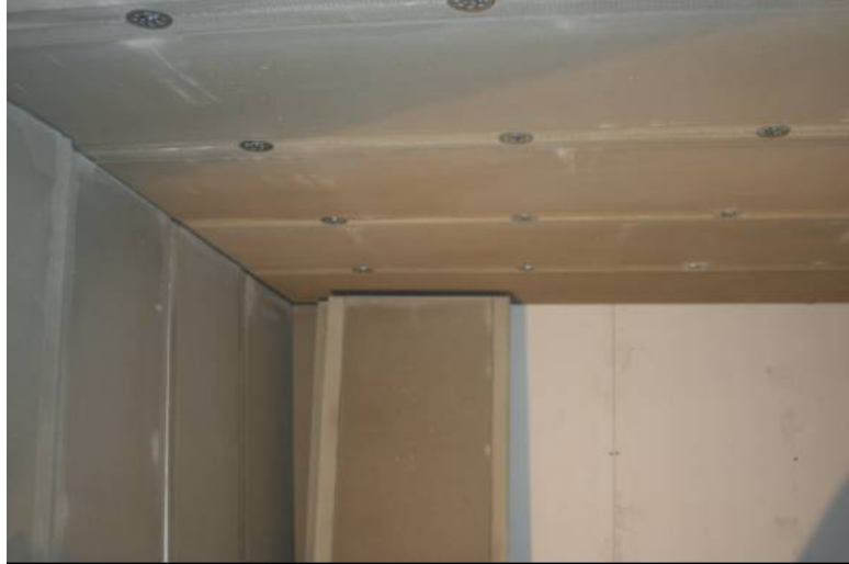
Figure 2. Ceiling Panels Installed, and Wall Panels Partially Installed.
