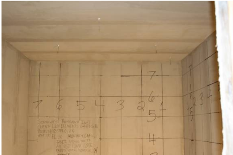
Figure 3. Pre-Test View of Completed Room.
