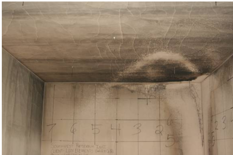
Figure 6. Post-Test View of Back Wall at Ceiling.
