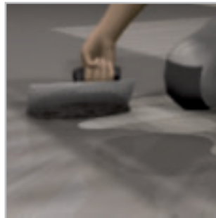
DRY-ASK – Filling wall and floor surfaces
