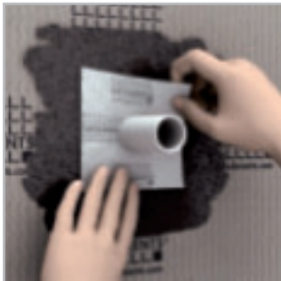
DRY-DBWM – Sealing pipe duct
