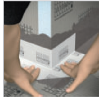
DRY-DB(V)AE – Forming exterior corners
