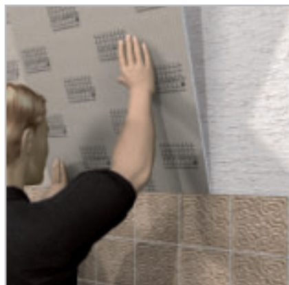
... application on walls (e.g. as wall levelling over existing tile coverings) ...
