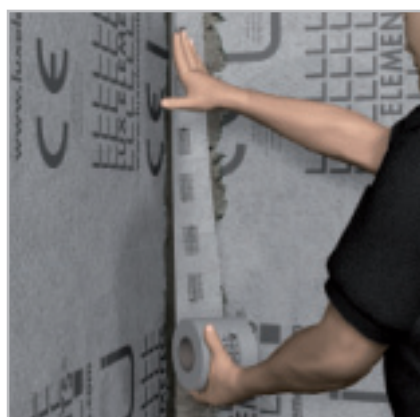
Sealing of the joints and corners using DRY-DBV
