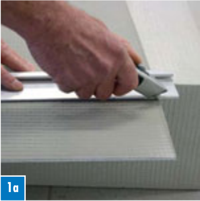
1a Carry out a continuous cut on the top side of the hard foam support element along an applied ruler using the cutter.
