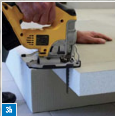
3b Before the actual cut, draw a cutting line using a pencil and a ruler. Then cut to size along the line using the jig saw (very easy cut).
