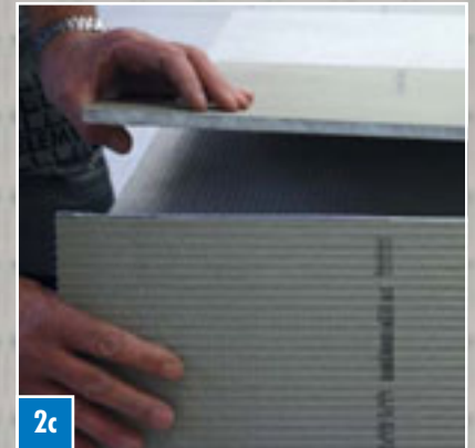
2c A smooth, clean cutting edge is created.
