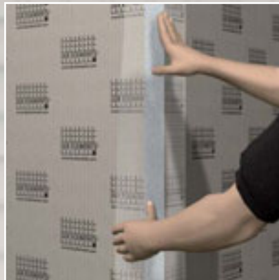
Slightly broader, self-adhesive reinforcement strips are used for the reinforcement of corners.
