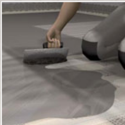
Liquid sealing compounds applied with a smoothing trowel are recommended for sealing hard foam support elements.
