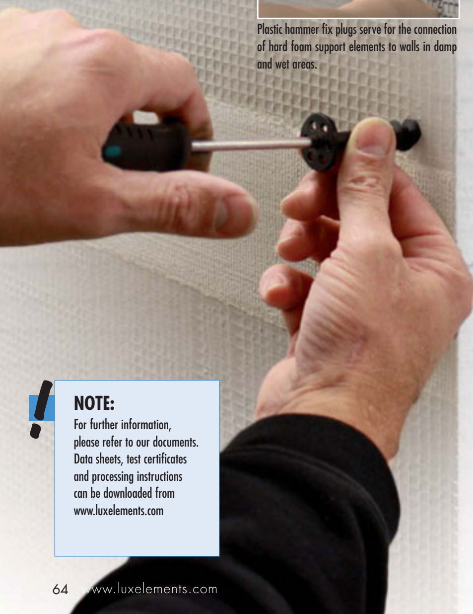
Plastic screw plugs enable the connection of hard foam support elements to one another.
