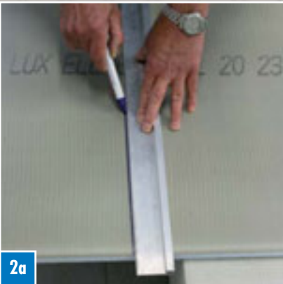
2a Before cutting, draw a cutting line using a pencil and a ruler.
