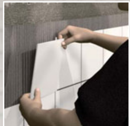
Tile laying using the thin-bed method. Apply tile adhesive over the full surface using a notched trowel.
