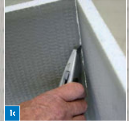
1c Then use the cutter to sever the mortar layer and the glassfibre fabric on the rear side of the hard foam support element in its bent state.
